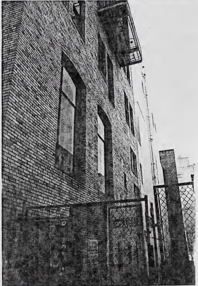
We went in over this fence to the fire escape.
